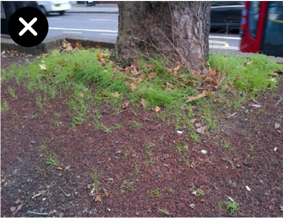
Poor example of rubber crumb application
