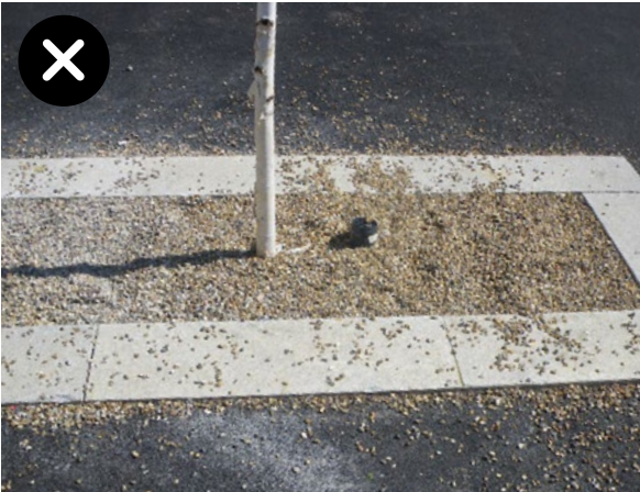
Poor example of inorganic mulch application
