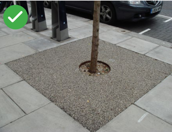
Good example of resin-bound gravel application
