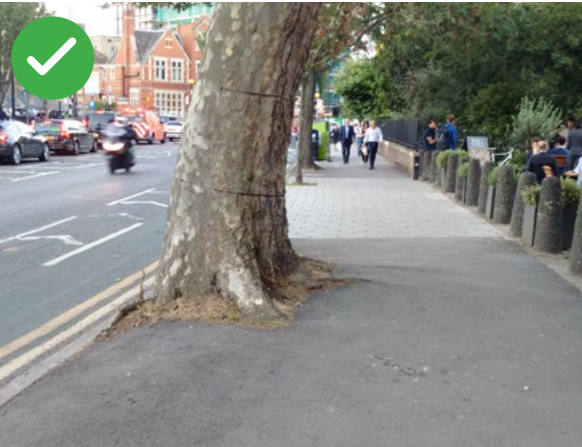
Good example of asphalt application
