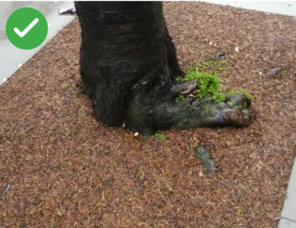
Good example of rubber crumb application
