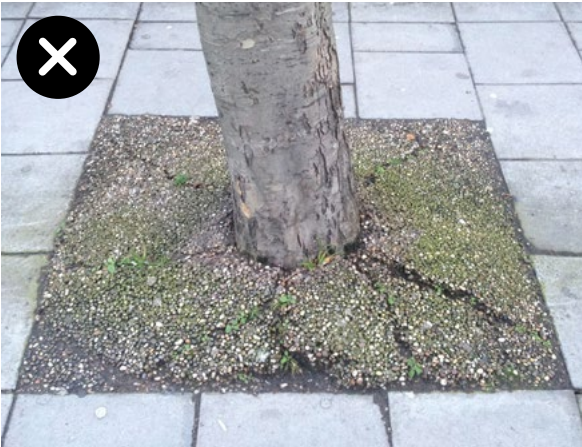
Poor example of resin-bound gravel application
