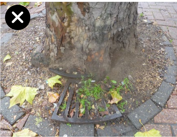
Poor example of grille application
